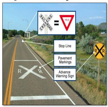
Figure 2.16 Railroad Crossing Pavement Markings
